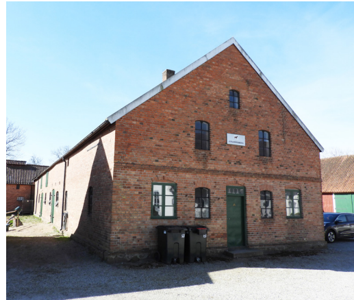
Kostallets gavel mot norr.
